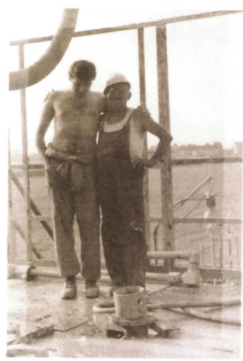
Figure 4- Personal protective equipment on the job floor 30 years ago
