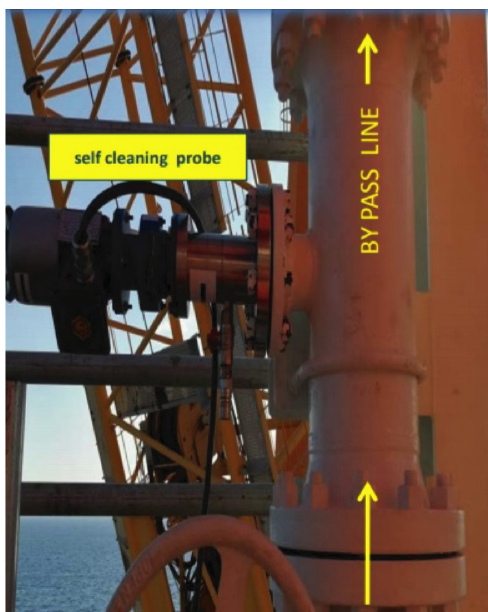
Fig.1: Self-cleaning probe installed on the 6" by-pass line
